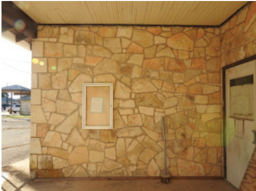
Figure 3.28: South face of recessed, covered entrance
