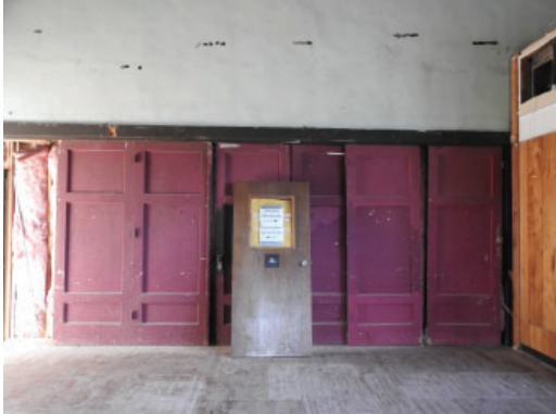
Figure 3.43: Sliding accordion door partition system
