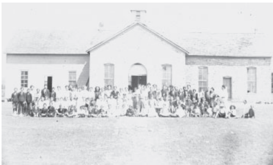
Figure 2.3: Dripping Springs Academy as a one story structure
