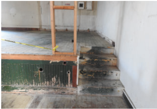
Figure 3.47: Stairs to stage. Note wood beadboard proscenium
