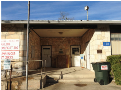
Figure 3.6: Recessed opening at the east elevation
