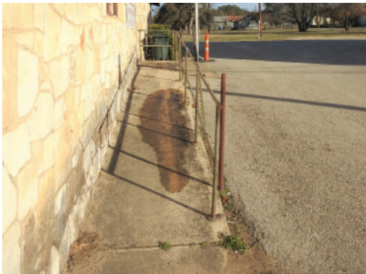
Figure 3.53: Ramp leading to concrete platform
