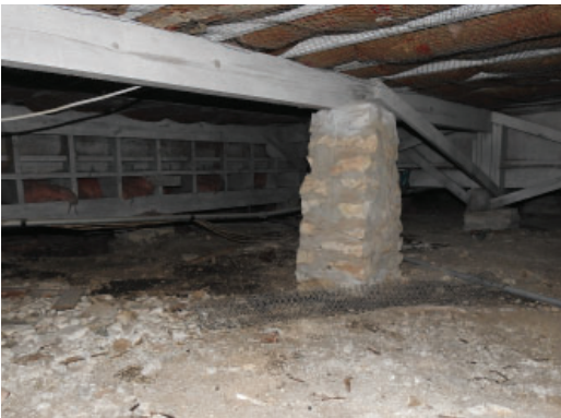
Figure 3.3: Limestone masonry foundation pier and wood beam structure in crawl space under stage at north end
