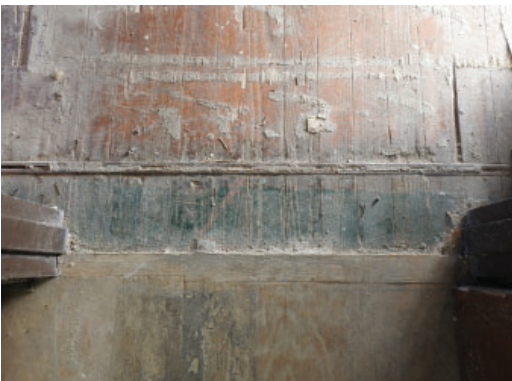
Figure 3.39: Threshold between remodeled space and main auditorium
