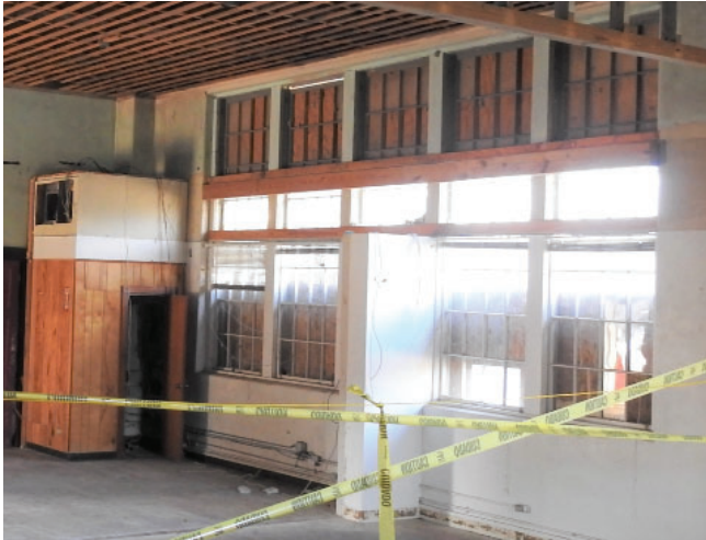
Figure 3.21: Interior with remnants of two dropped ceilings over windows
