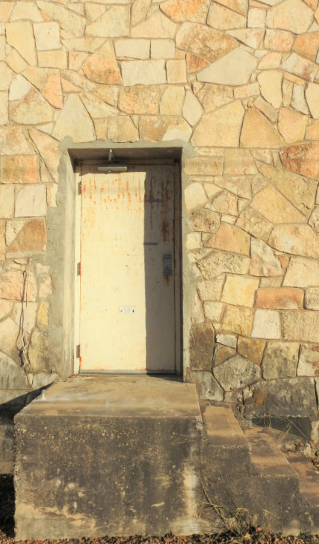
Figure 3.24: Non-original hollow metal door in non-original masonry opening
