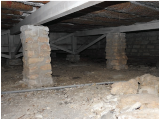
Figure 3.2: Limestone masonry pier and wood beam structure
