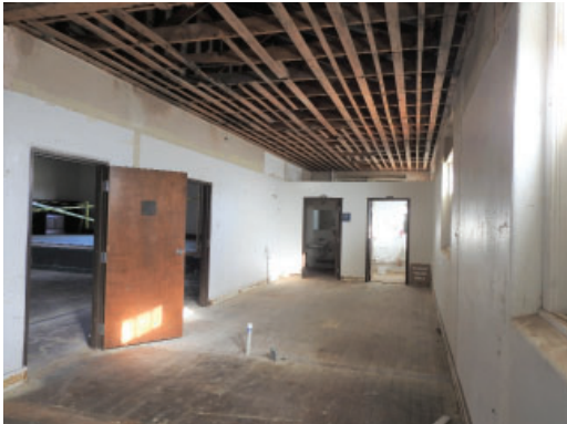
Figure 3.35: Classroom with non-original restrooms built at back of room
