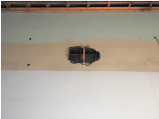
Figure 3.34: Original interior wall. Note three paint colors, signifying the addition of two dropped ceilings
