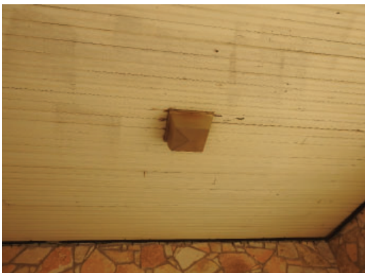
Figure 3.30: Ceiling and light fixture of recessed, covered entrance
