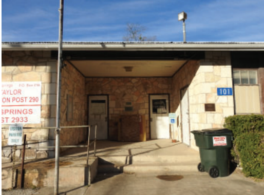
Figure 3.27: Recessed, covered entrance on east elevation
