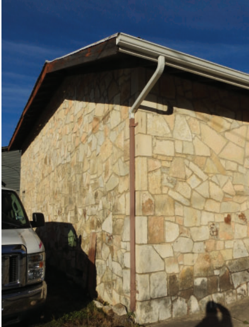
Figure 3.31: Single metal gutter at southeast corner
