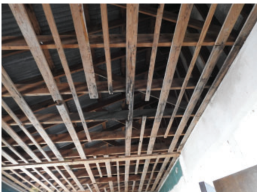
Figure 3.12: Wood trusses visible through ceiling
