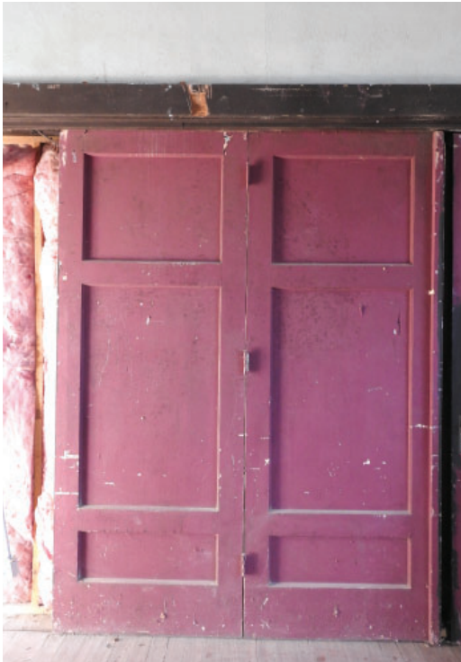
Figure 3.44: Three panel wood doors with original hardware
