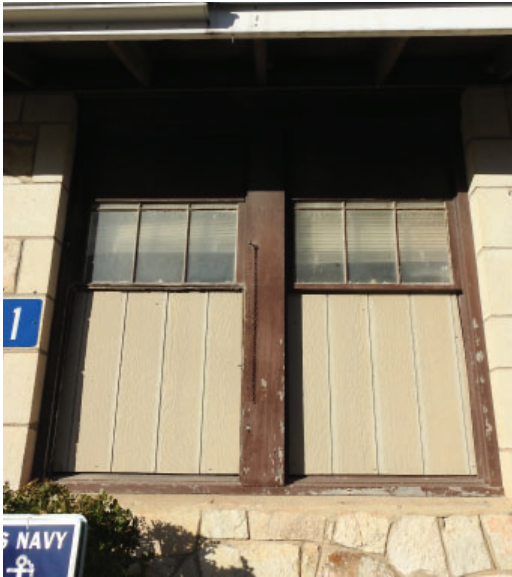
Figure 3.13: Typical double-hung window pair, lower panes boarded-over from exterior.
