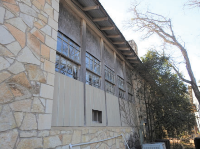
Figure 3.19: Set of 5 double-hung, 16-over-16 lite windows on west elevation
