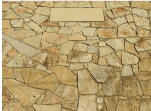
Figure 3.5: Exterior rough cut limestone masonry with V-groove mortar detail
