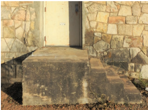
Figure 3.54: Concrete steps up to entrance landing
