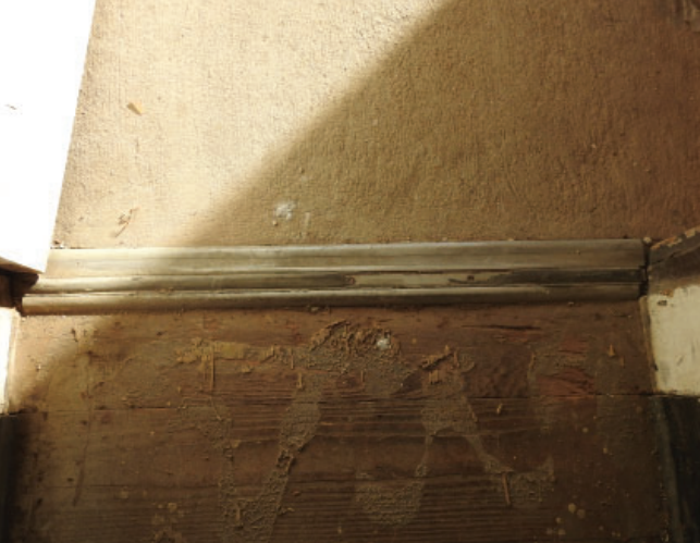
Figure 3.25: Typical metal threshold at front entry
